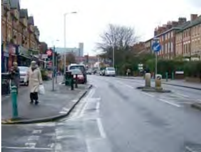
This juxtaposition of this central island and oversized build-out produce a space conflict that makes a mockery of the preceding short length of cycle lane.
