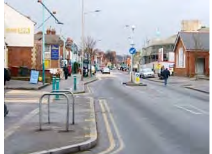
Locating this crossing island next to the build out at the bus stop creates a pinch point.
