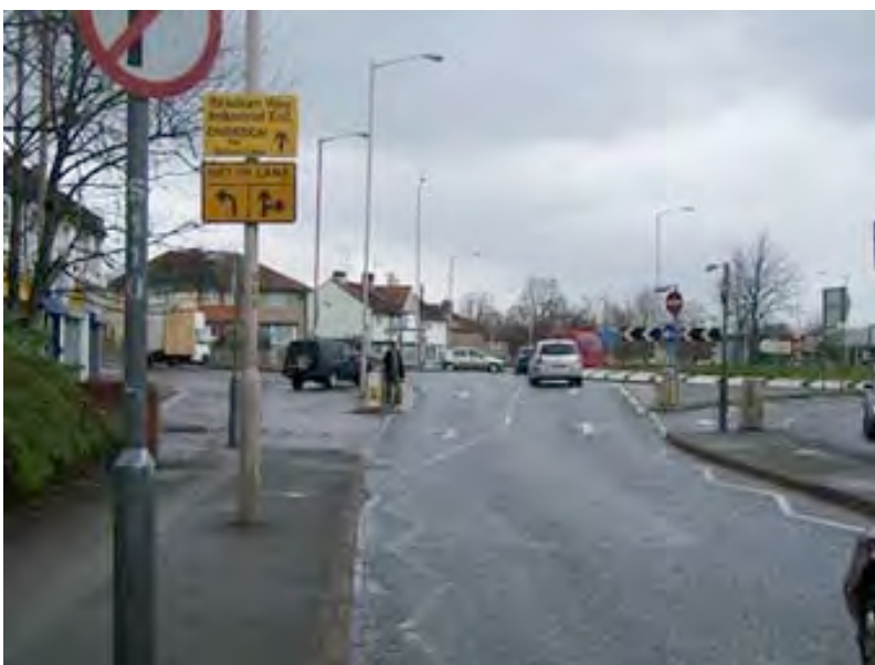
The westward approach to Norcot roundabout would be easier for cyclists if the left lane were not a dedicated left turn. This recent traffic measure has made the roundabout more treacherous for cyclists.
